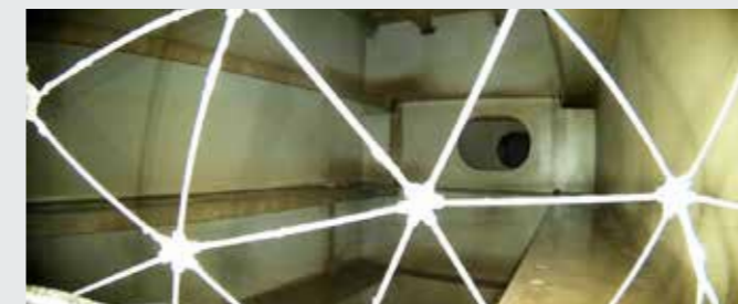
General Visual Inspection
