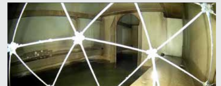
General Visual Inspection
