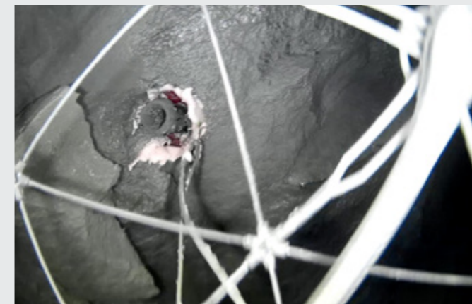
DRILLING HOLE WITH EXPLOSIVE EMULSION LEFT
