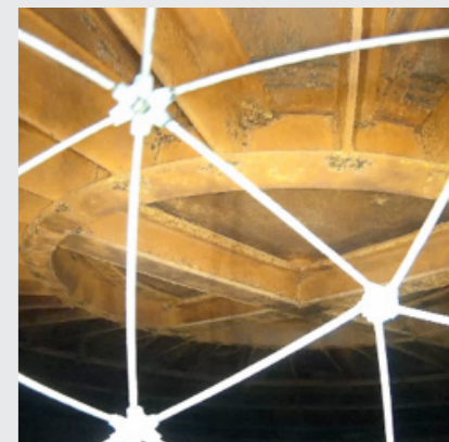
Roof visual inspection
